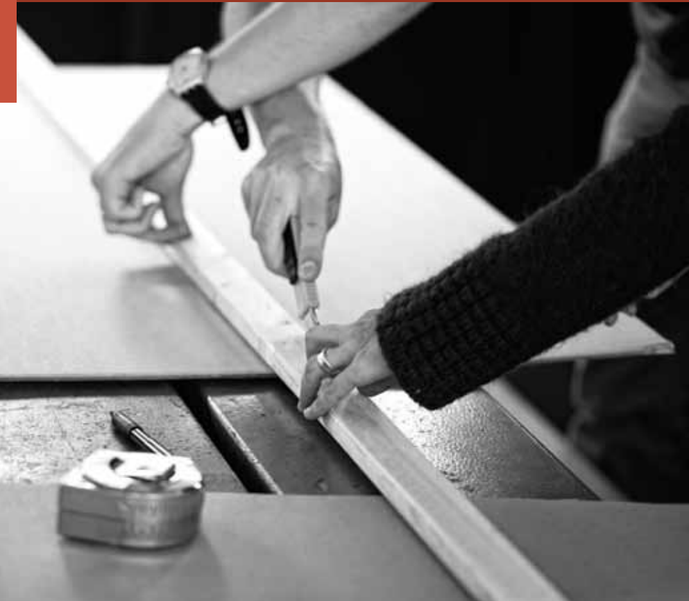
▲ Sheets of cardboard are cut to line the camper's interior.
